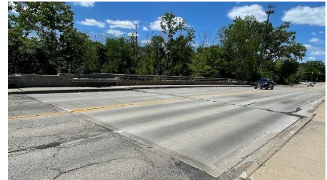
General View of Bridge (Looking West)
